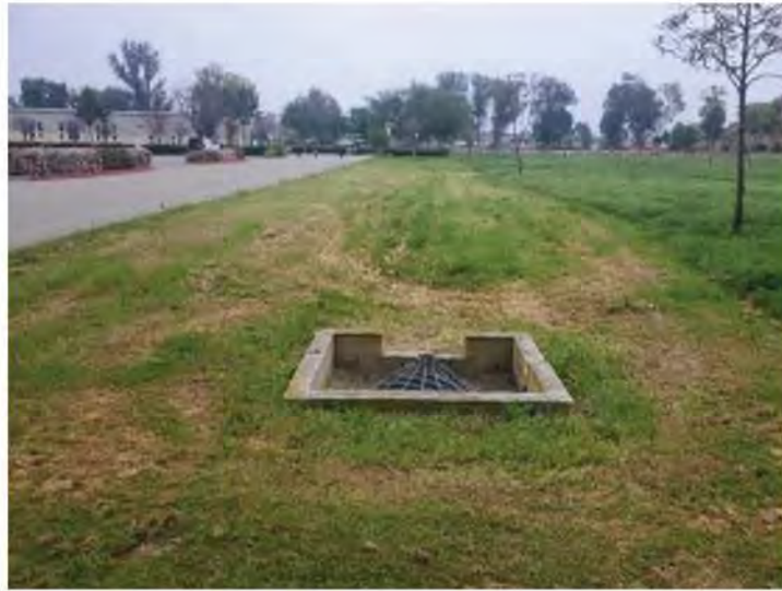
Photograph 7: View of typical storm drain on the subject property.
