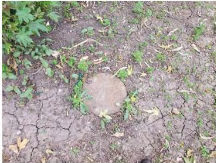
Photograph 9: Close up view of potential well cover on the subject property.
