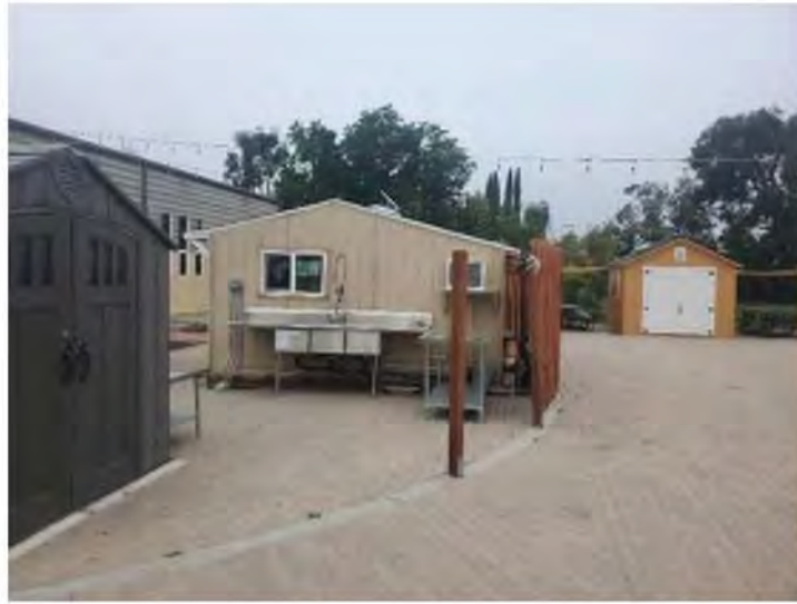
Photograph 3: View of additional outbuildings north of the church on the subject property.
