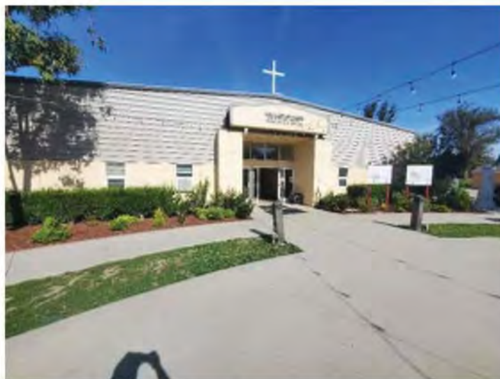
Photograph 1: View of subject property building looking south.
