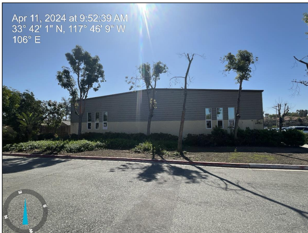
Looking east at the main church building.
