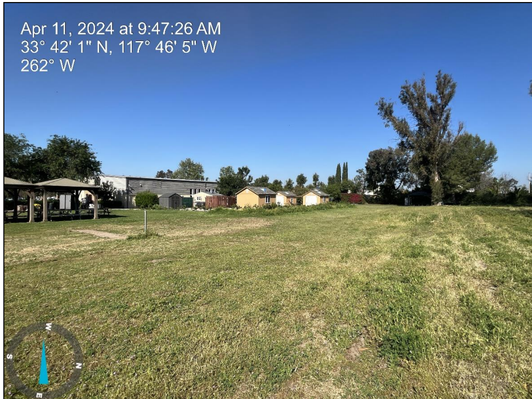
Looks west at the main building and accessory buildings.
