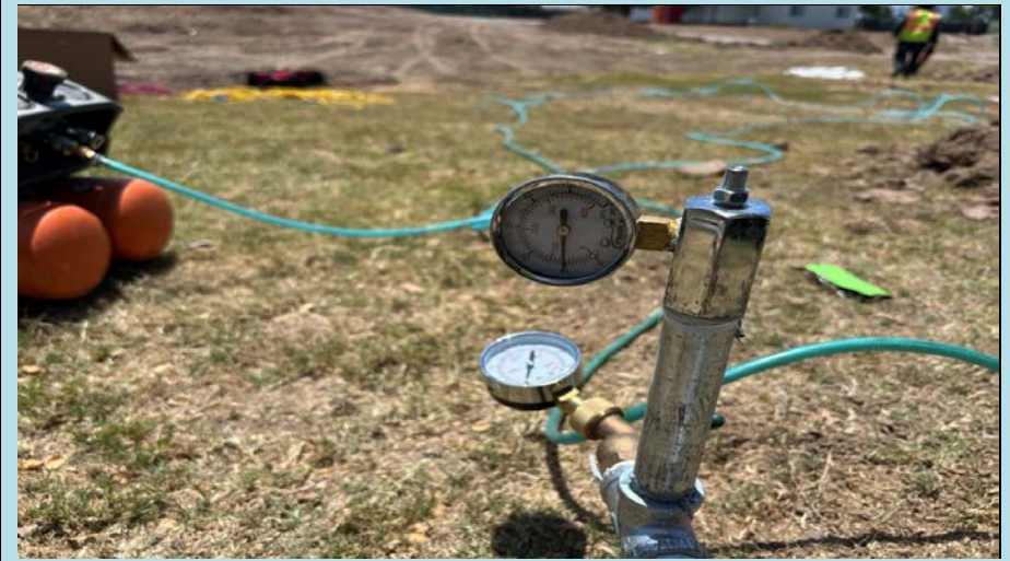
High-Line pressure tested for leak detection
