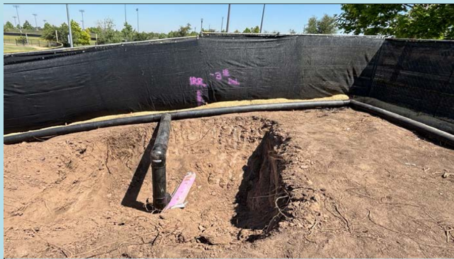
elbows added to highline for connections to existing irrigation lines
