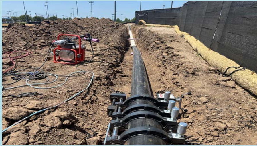
Ongoing high-line installation, including sleeve under future driveway
