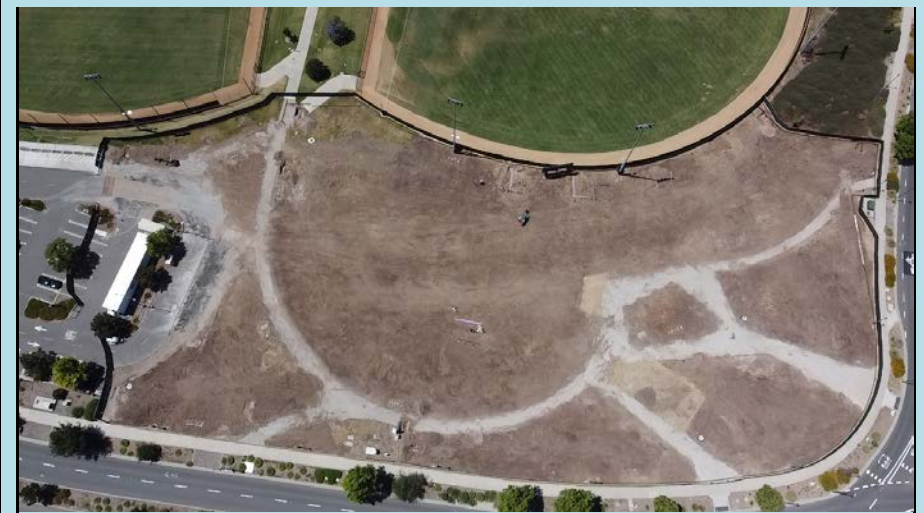
Aerial view of progress at job site
